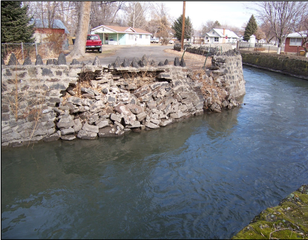
Figure 22. Parapet walls prevent reconnection to the local floodplain.
