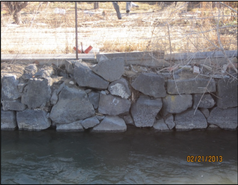
Figure 7. A section of the channel wall constructed of stacked, ungrouted rock.
