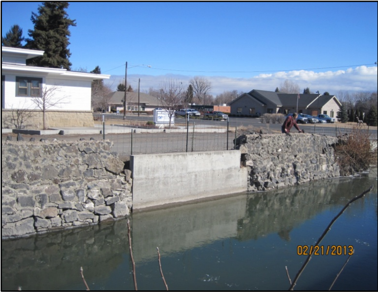
Figure 15. New concrete wall replacement (accomplished during the 1990s)
