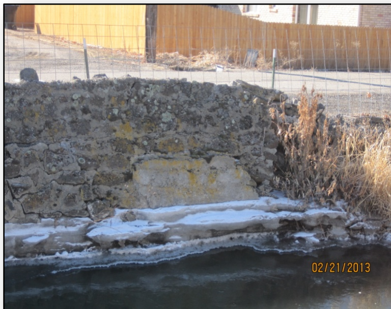
Figure 13. Concrete used to repair channel wall section.
