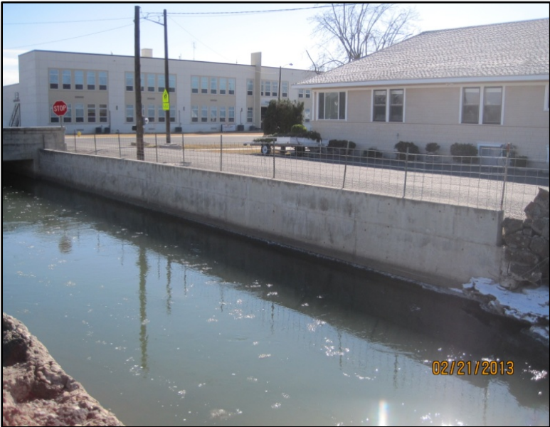
Figure 14. New concrete wall replacement (accomplished during the 1990s)
