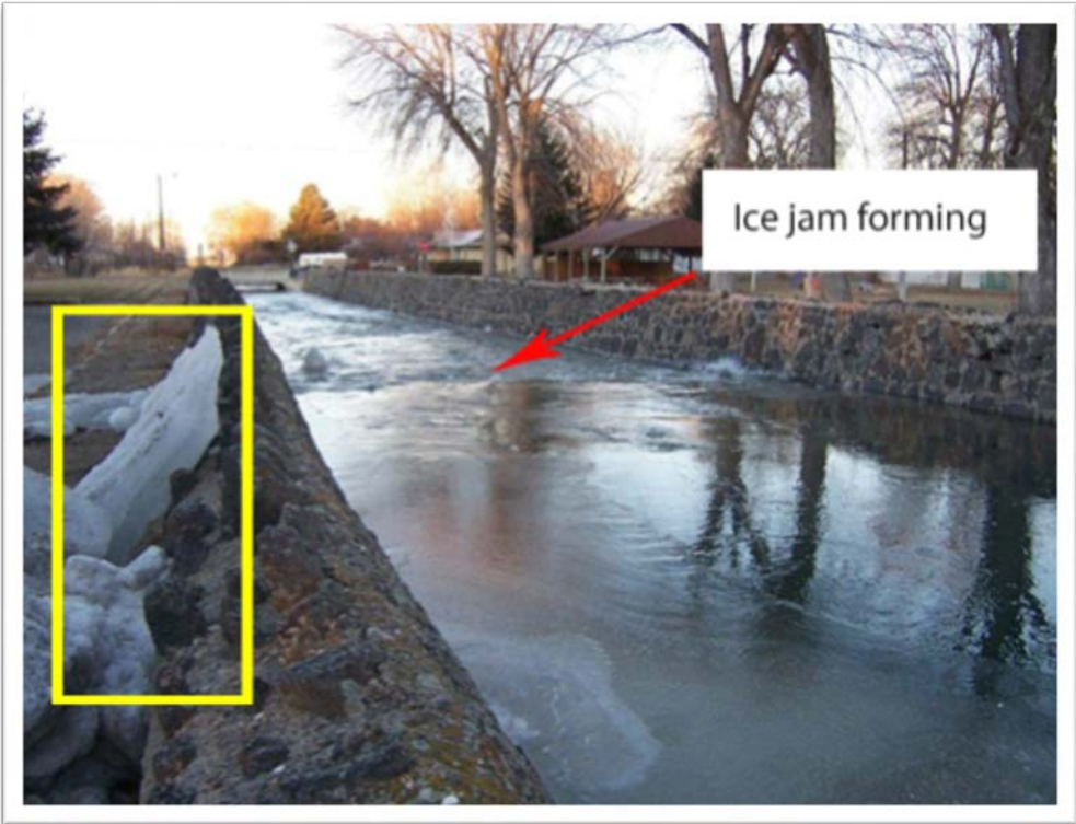
Figure 19. Ice jam upstream of Nevada Street Bridge. Removed ice is visible on the left.
