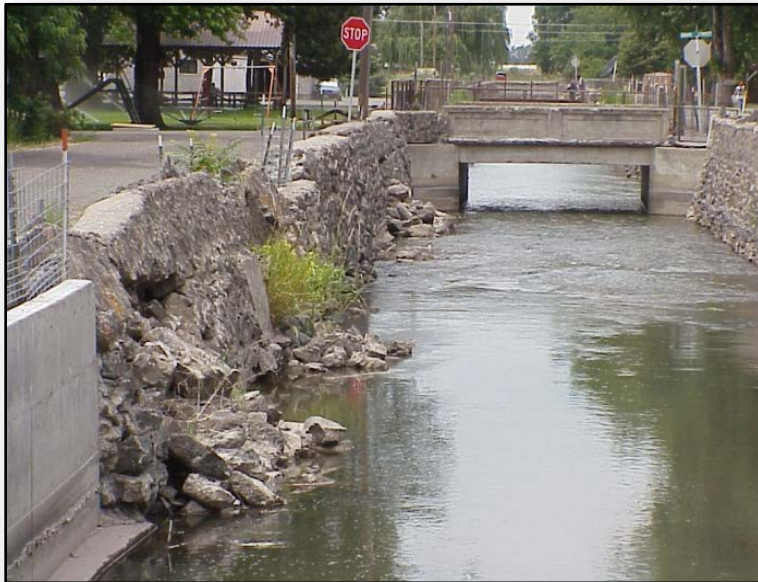
Figure 1. Typical section of the Gooding Canal with stones sloughing into channel and narrow bridges constricting flow.
