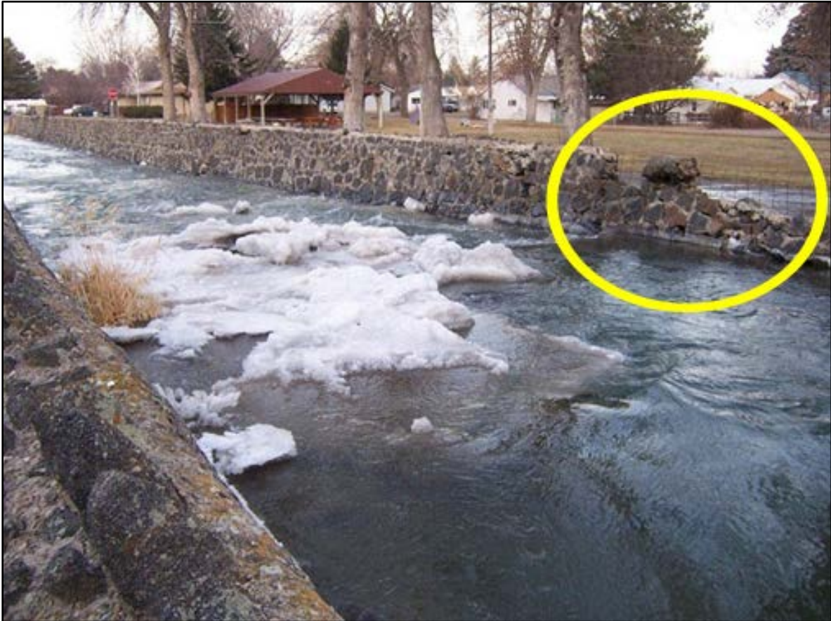
Figure 20. Ice jam upstream of Nevada Street Bridge. Water has escaped the channel and caused localized flooding in the city park.
