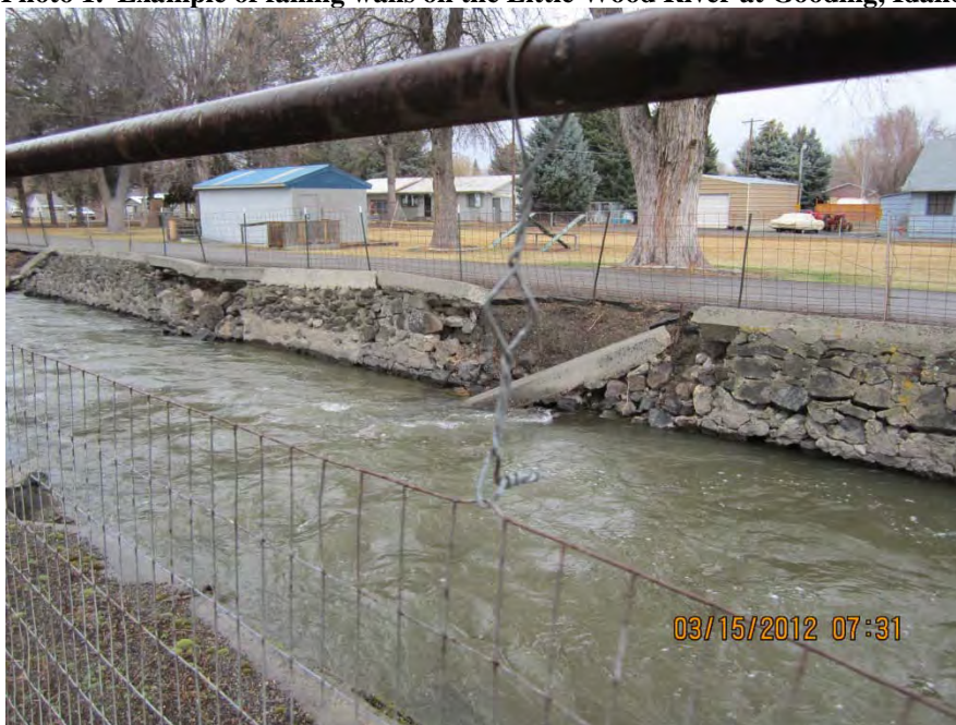
Photo 1. Example of failing walls on the Little Wood River at Gooding, Idaho.
