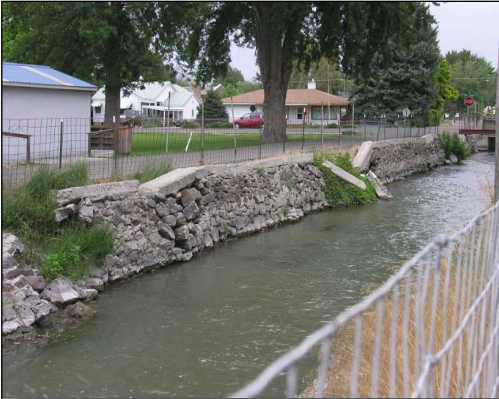
Figure 21. Failing walls contribute to damage to adjacent infrastructure.
