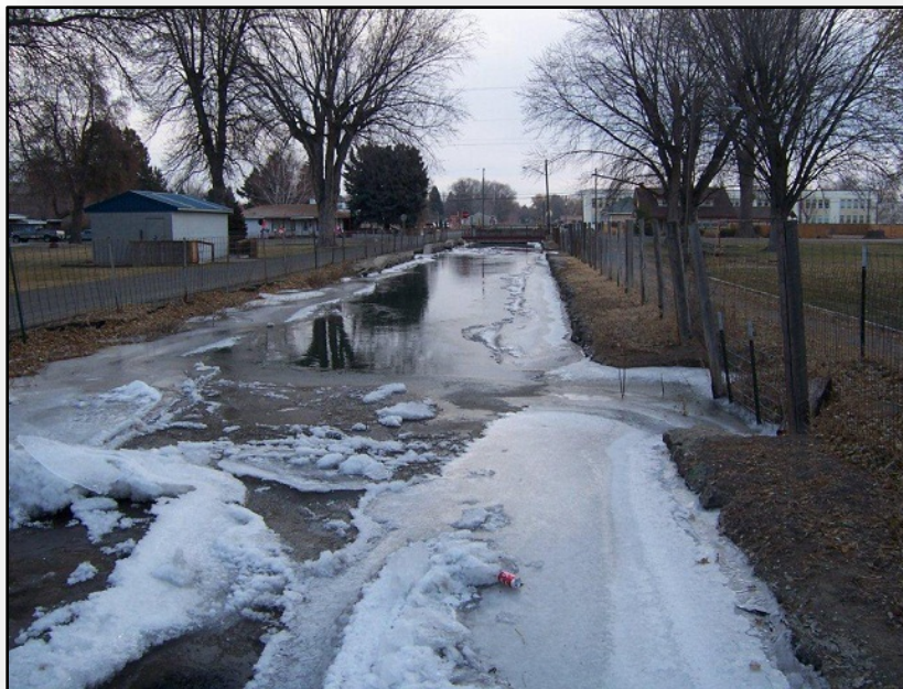
Figure 10. Ice jam forming in-between the Nevada and Idaho Street bridges.
