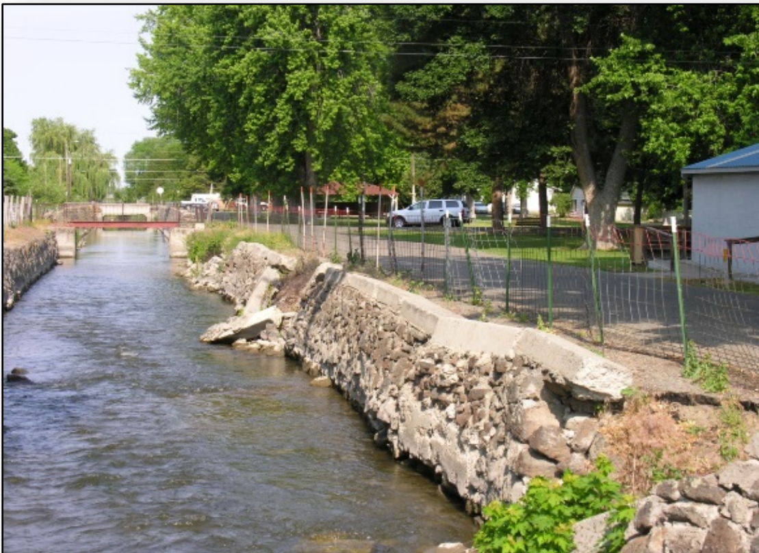
Figure 18. Collapsed wall sections, despite attempts to stabilize with concrete capping.
